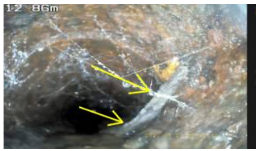
Photo 3-2 looks like a rag or towel of some sort. Recommend Cleaning Line
